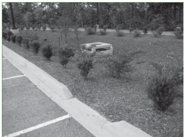
Parking lot runoff treated by bioretention
